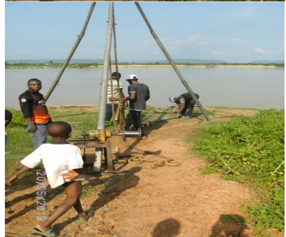
Plate 2: Collection of soil samples and different depth using Bucket Auger
